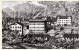
Fabrikansicht 1880 View of the factory 1880
