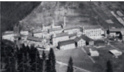
Fabrikansicht 1898 View of the factory 1898
